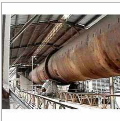
Cement Plant Inspection
