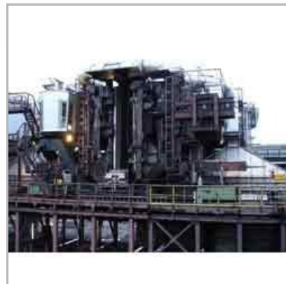
Inspection Of Coke Oven Machine
