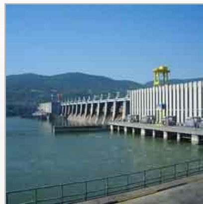
Inspection Of Hydraulic Power Plant
