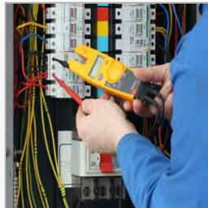
Civil & Electrical Inspection
