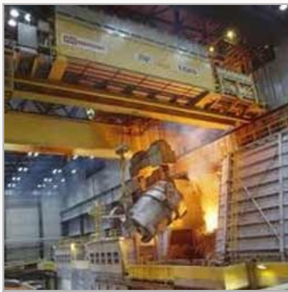
Inspection Of EOT Cranes
