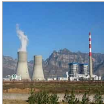
Turnkey Projects Of Thermal Power Plant
